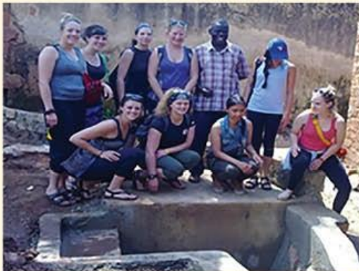
Construction of a spring well
